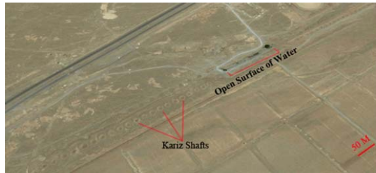
Figure 6. Hassan-Abad's Kariz with chain of wells (from Google earth). Open surface of water (canal) and wells pattern.
